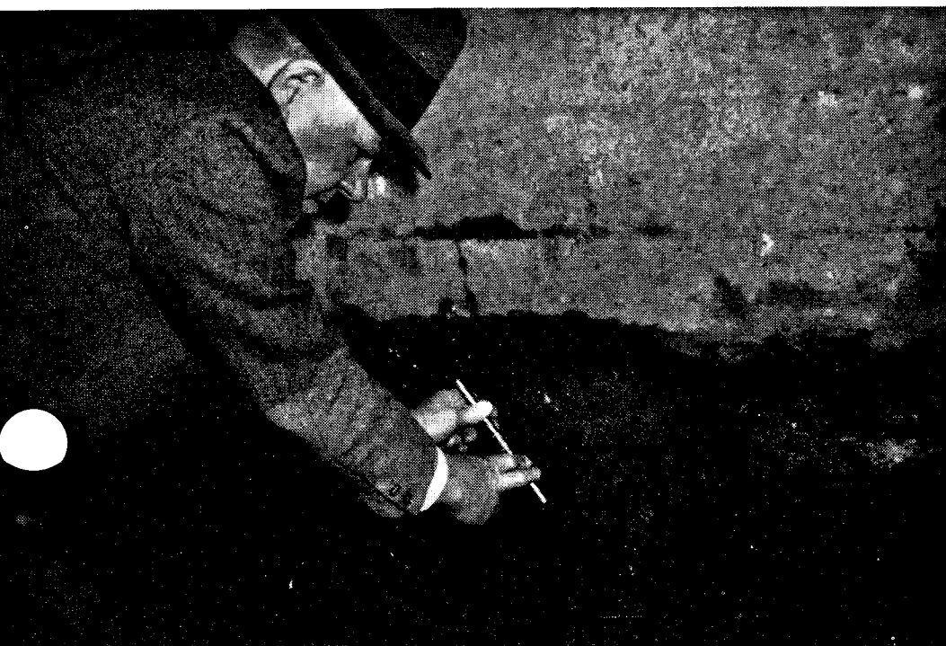
AWPI Senior District Engineer Ralph H. Mann, at the site of the 1939 Perisphere, New York World's Fair, is shown taking an increment boring from one of three piles at a point about 10 in. below bottom face of concrete base slab which rests upon the pressure-creosoted piles. Tops of the piles extend about 3 ft. above permanent ground water level.
