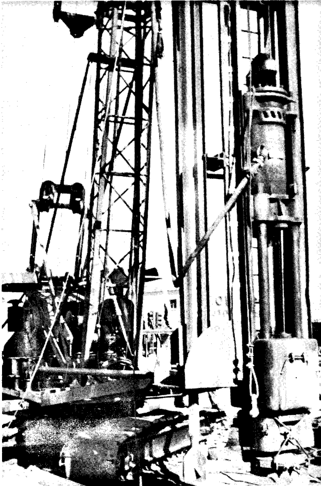
Fishtail bit mounted on side of pile driver leads. Power is supplied from the crane to the turntable of the drill. Drill is 12 inches in diameter and comprises four prongs.
